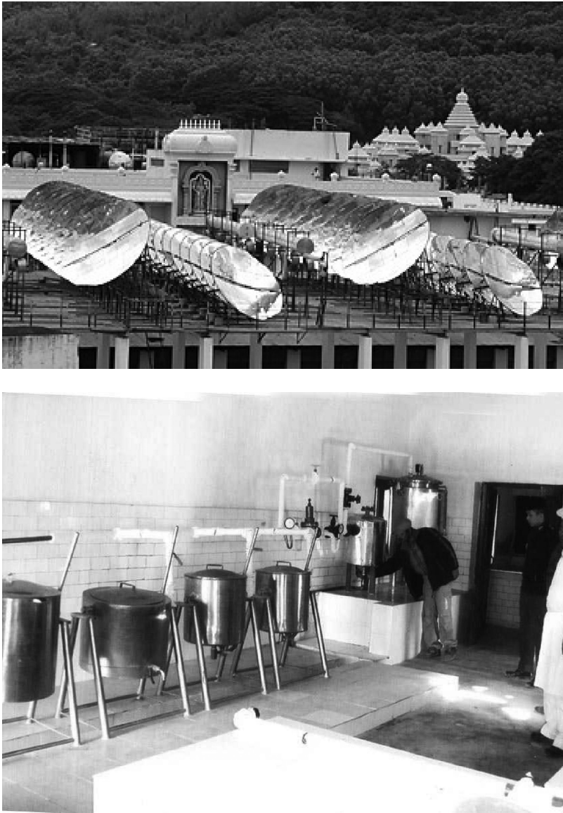
Figure 2. Solar Collectors Installed in a Religious Center (top) and a Typical Kitchen Setup for Utilizing Steam for Cooking Purposes (bottom). Reprinted with permission.
